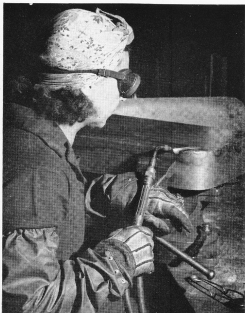
Bernice Knickerbocker, a trainee in the new Welding Shop, is fusing light-gauge steel together on a metal guard. The corners of the parent metal are joined by the heat of an oxy-acetylene torch.
