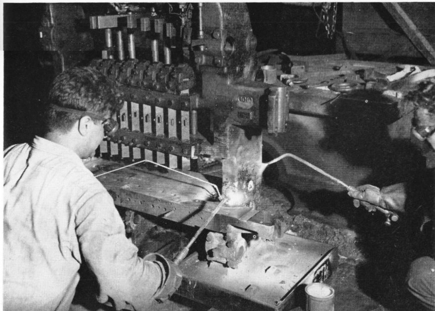
Charles Monterose, who served his apprenticeship at Scovill, is bronze-welding a cast-iron frame of an Eyelet machine. Henry Lubesky, an apprentice (to the right of the picture) is pre-heating the parent metal. This is necessary in order to prevent fatal changes in metal of the frame. The welding rods are made at Scovill.
